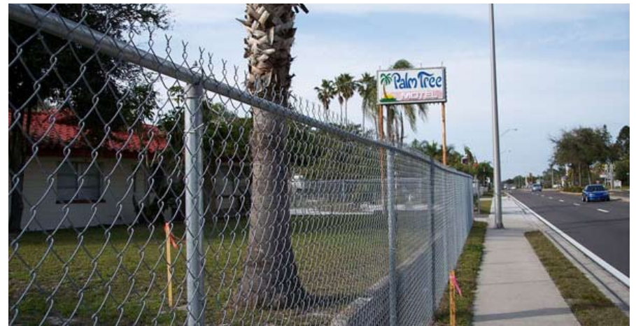
FIGURE 2: US 41 EXISTING CONDITIONS
